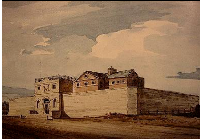
Bedford County Gaol and Old House of Correction c. 1820
